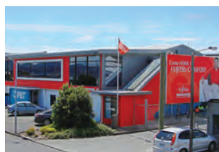
Fujitsu General New Zealand Ltd. (Nowa Zelandia)
