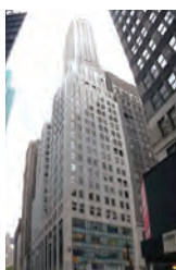
THE AIRSTAGE ON BROADWAY Fujitsu General Solution Center
