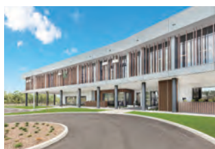
Fujitsu General (Aust.) Pty Ltd. (Australia)
